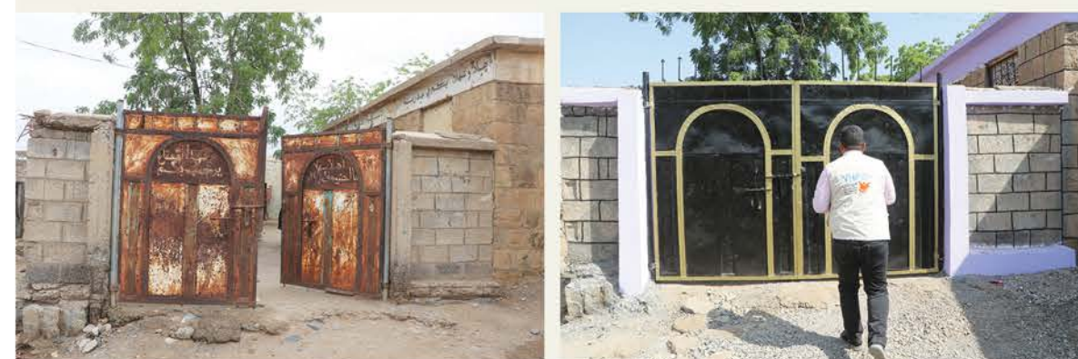
The school before rehabilitation
