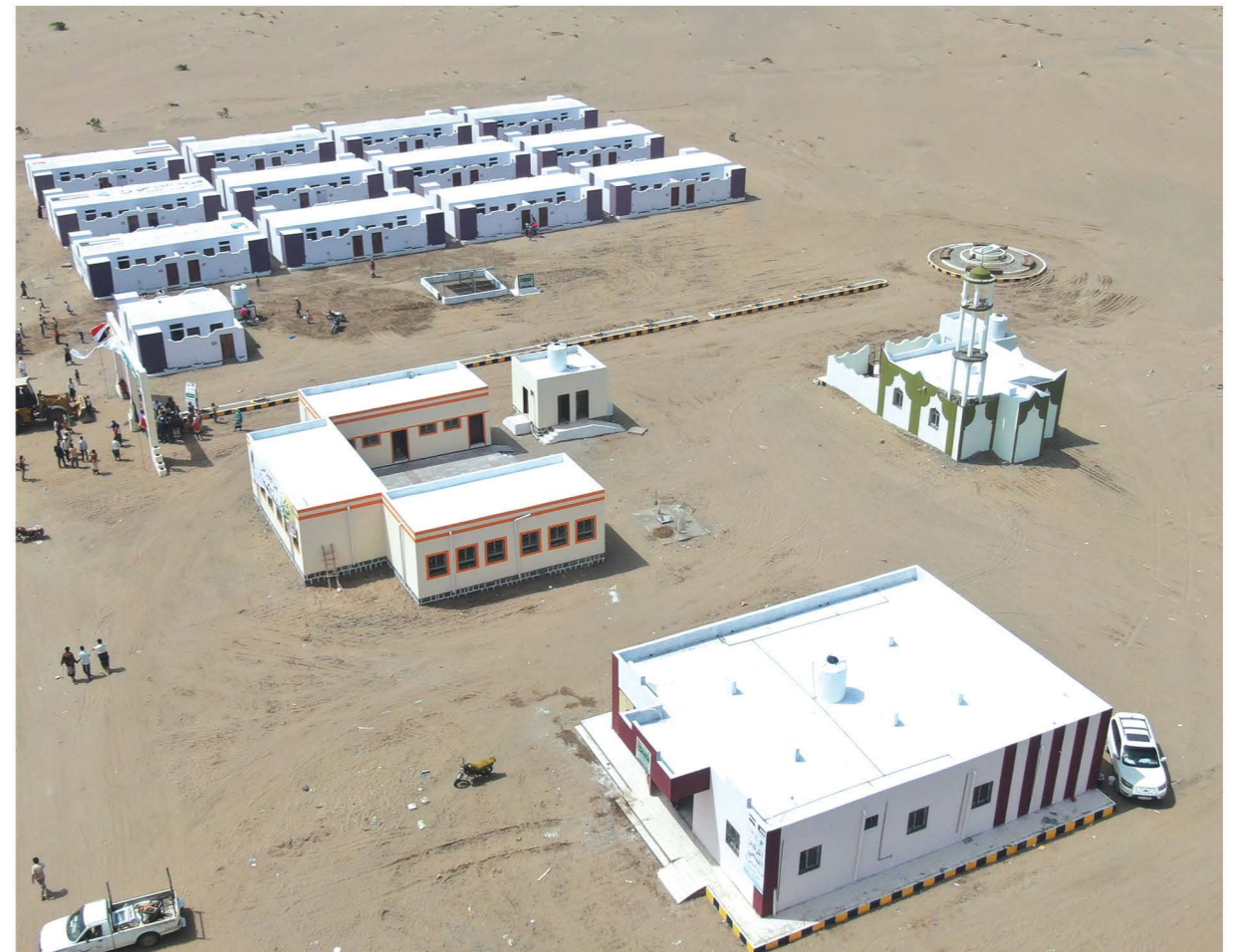
Al-Takhi Residential Village for IDPs shelter - Al-Khokha District - Al-Hodeidah Governorate
